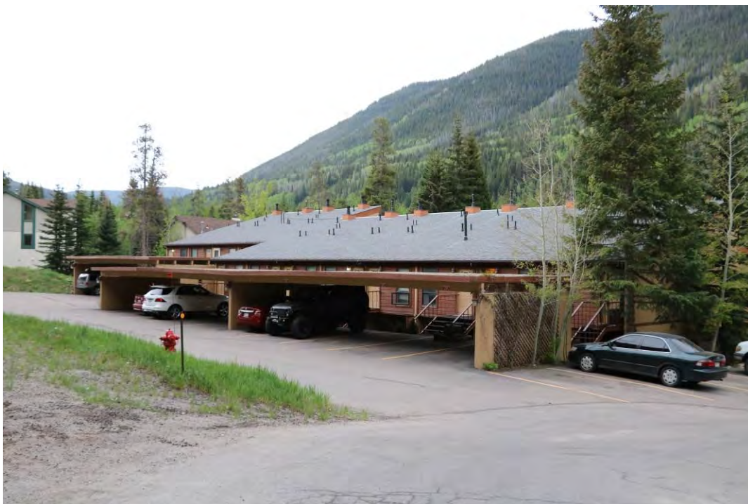
Overview of complex, view facing southeast.
