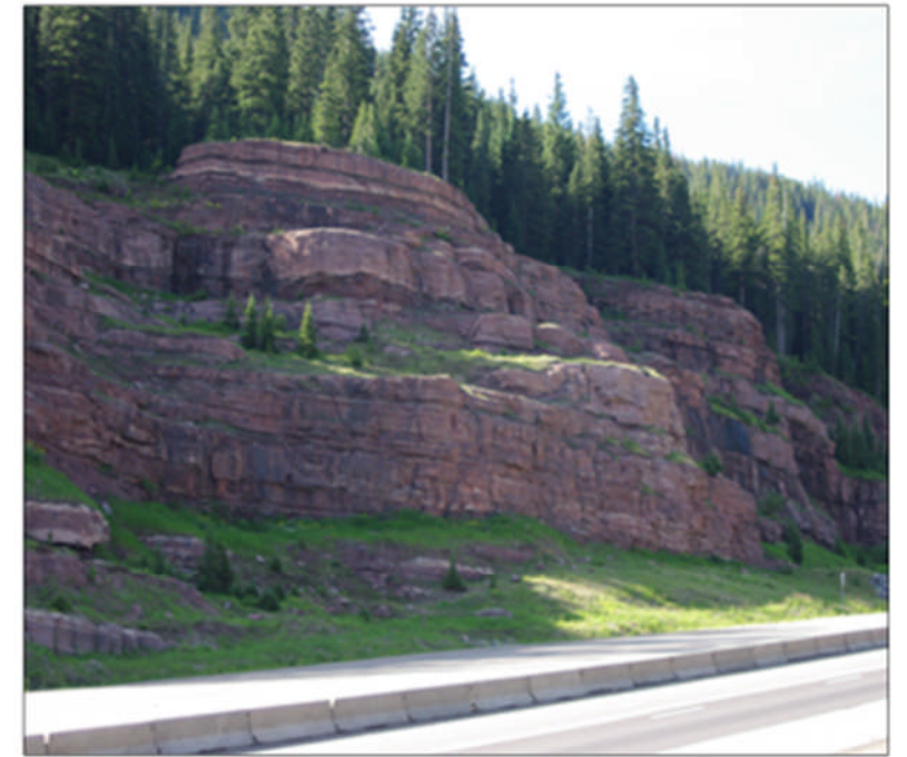
B | Rock cuts should include natural benches to mimic the surrounding landscape.
