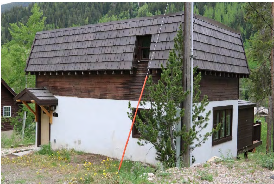
Overview of northeast (front) elevation and side (northwest) elevation with replacement wood deck and storage building visible at right, view facing south.
