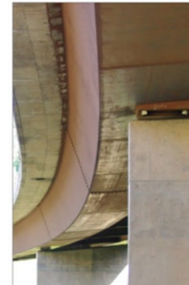
D | Use of accent color on bridge substructure.
