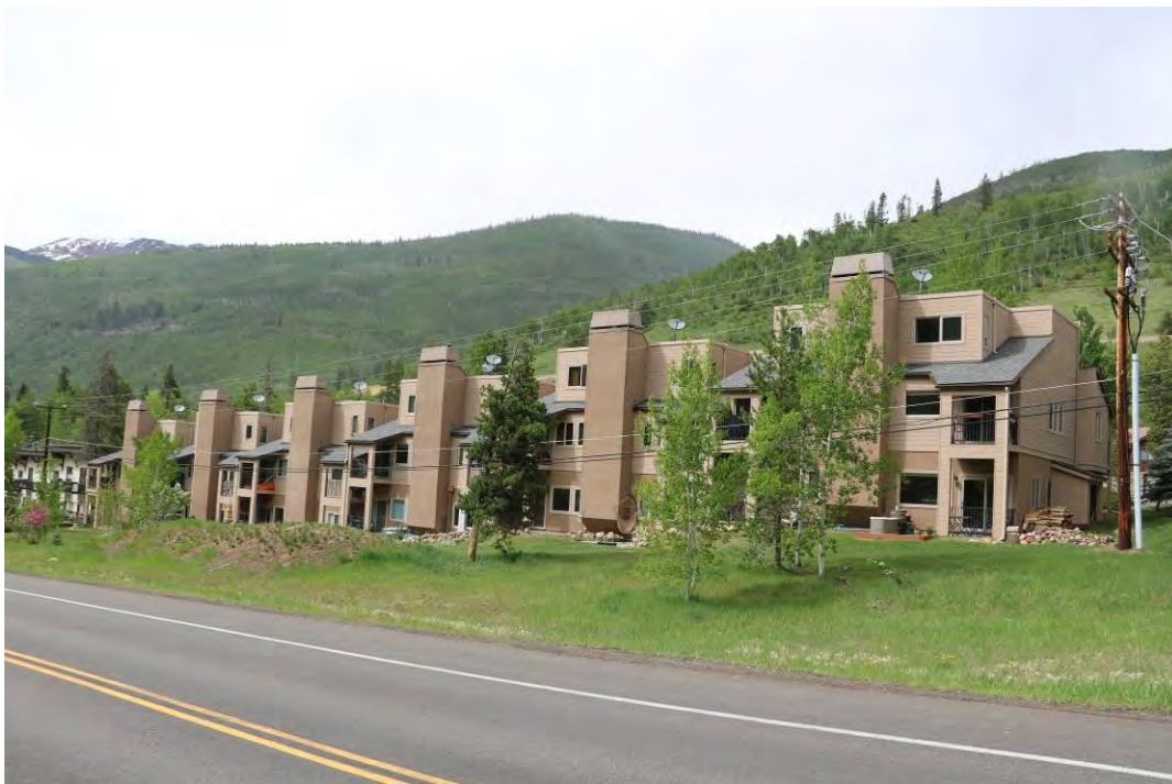
Overview of southwest (front) elevation and setting, view facing north.
