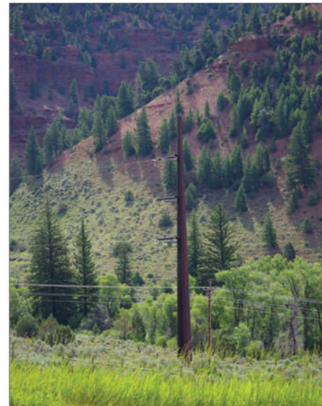
B / Proper color application based on the surrounding natural context blends utility structures
