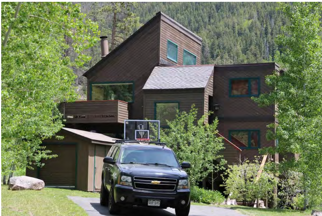
The front (northwest) elevation, view facing east.
