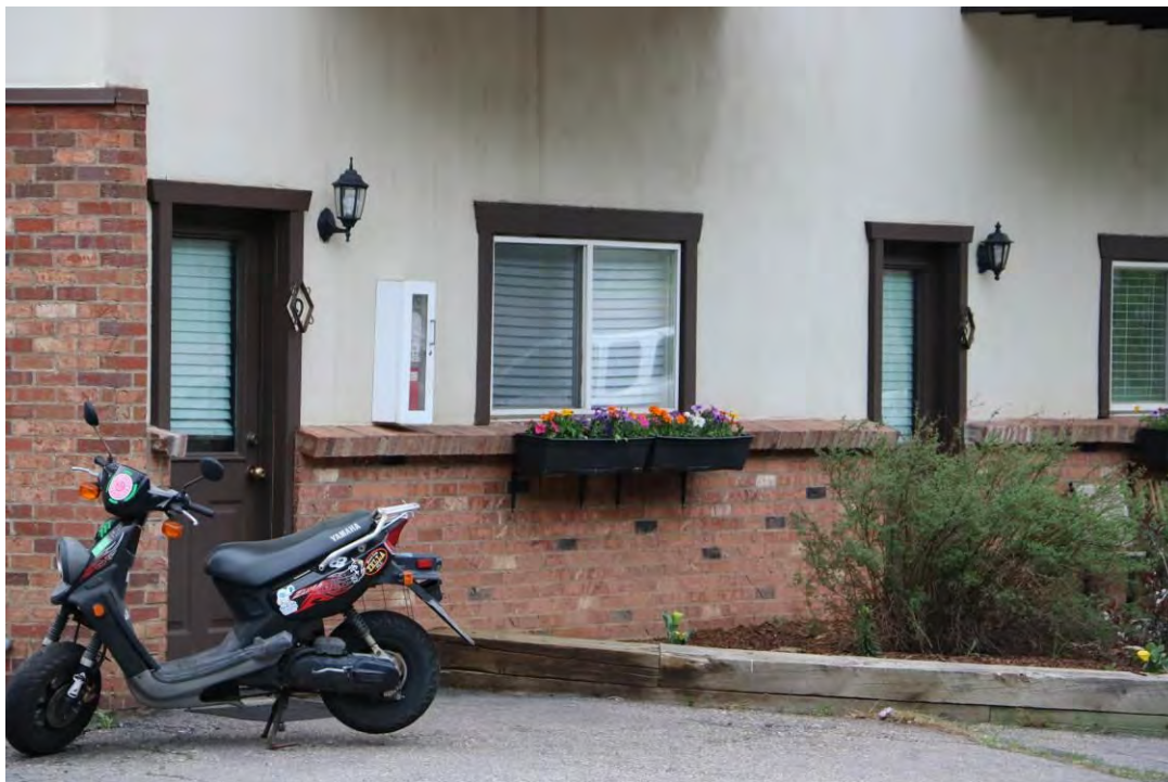
Detail of entryways on front (south) elevation, view facing northwest.
