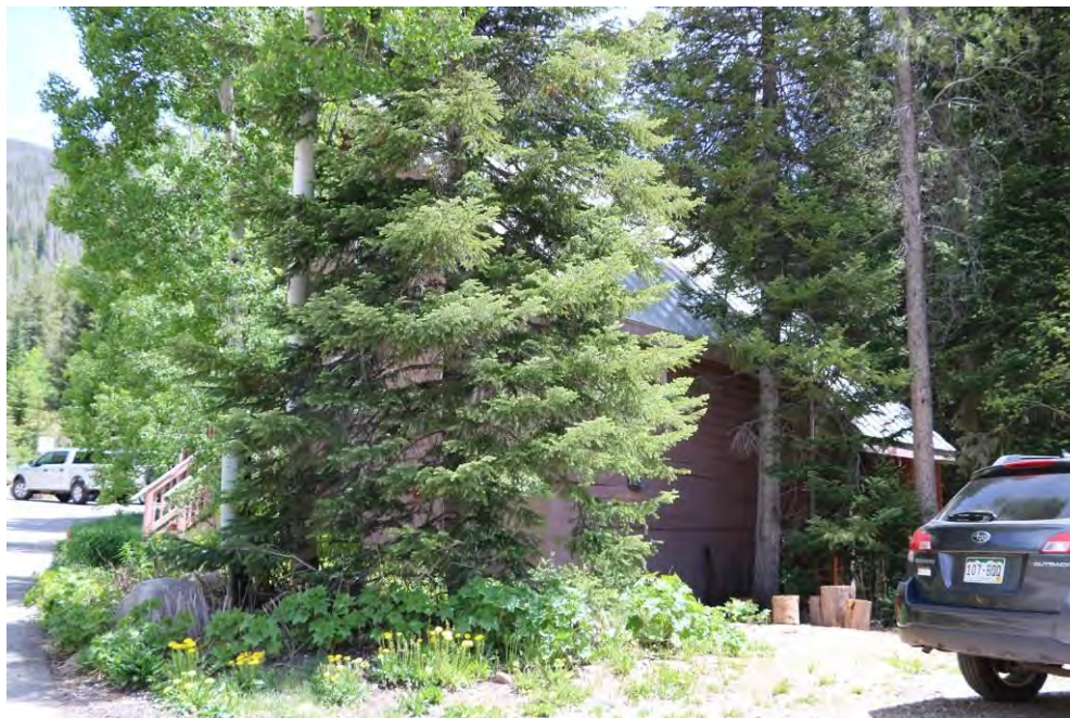
Side (southwest) elevation, view facing northeast.
