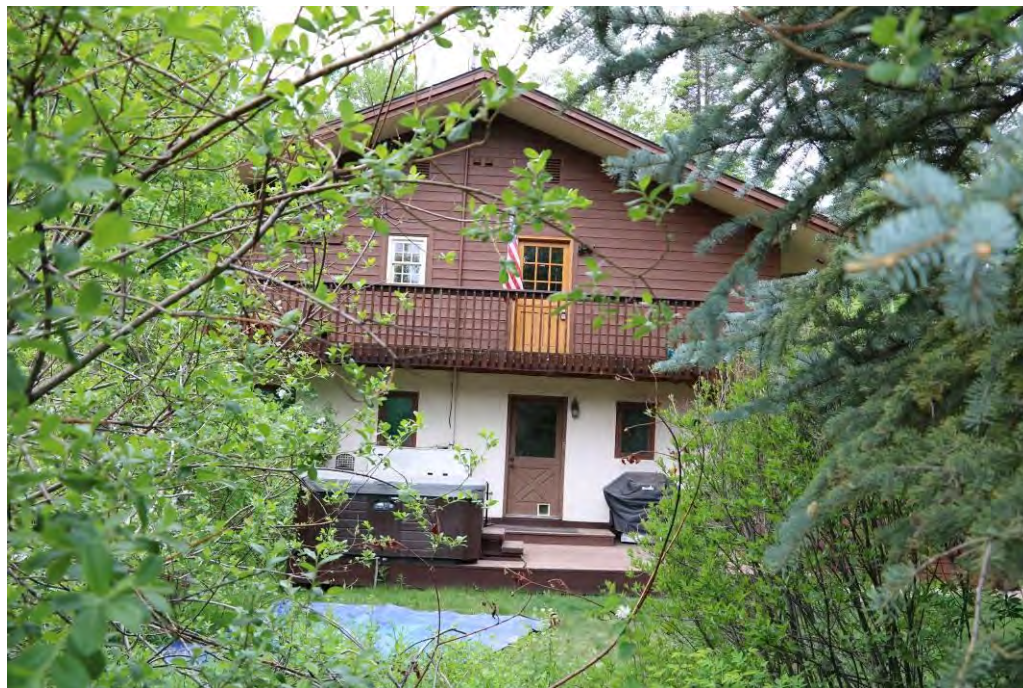
Front (east) elevation, view facing west.
