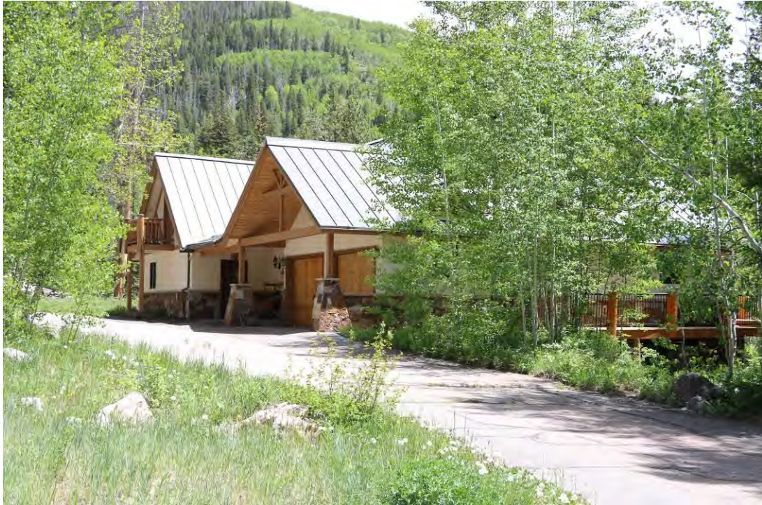
The front (north) and side (west) elevations, view facing southeast.
