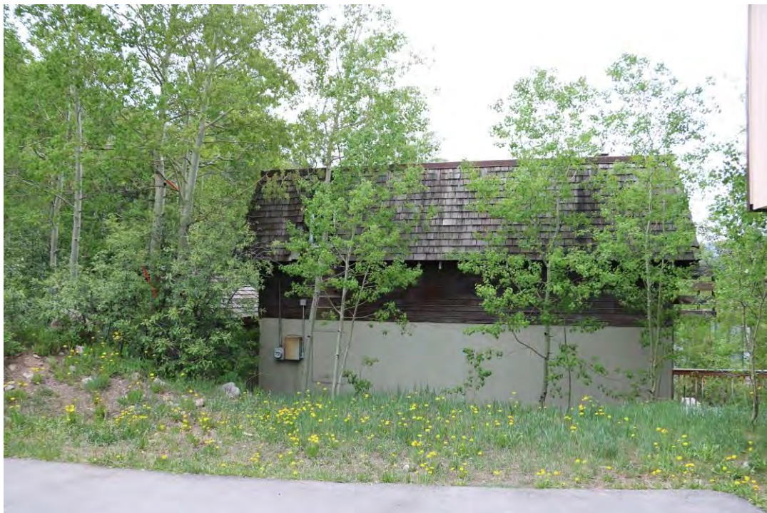
The side (northwest) elevation, view facing east.
