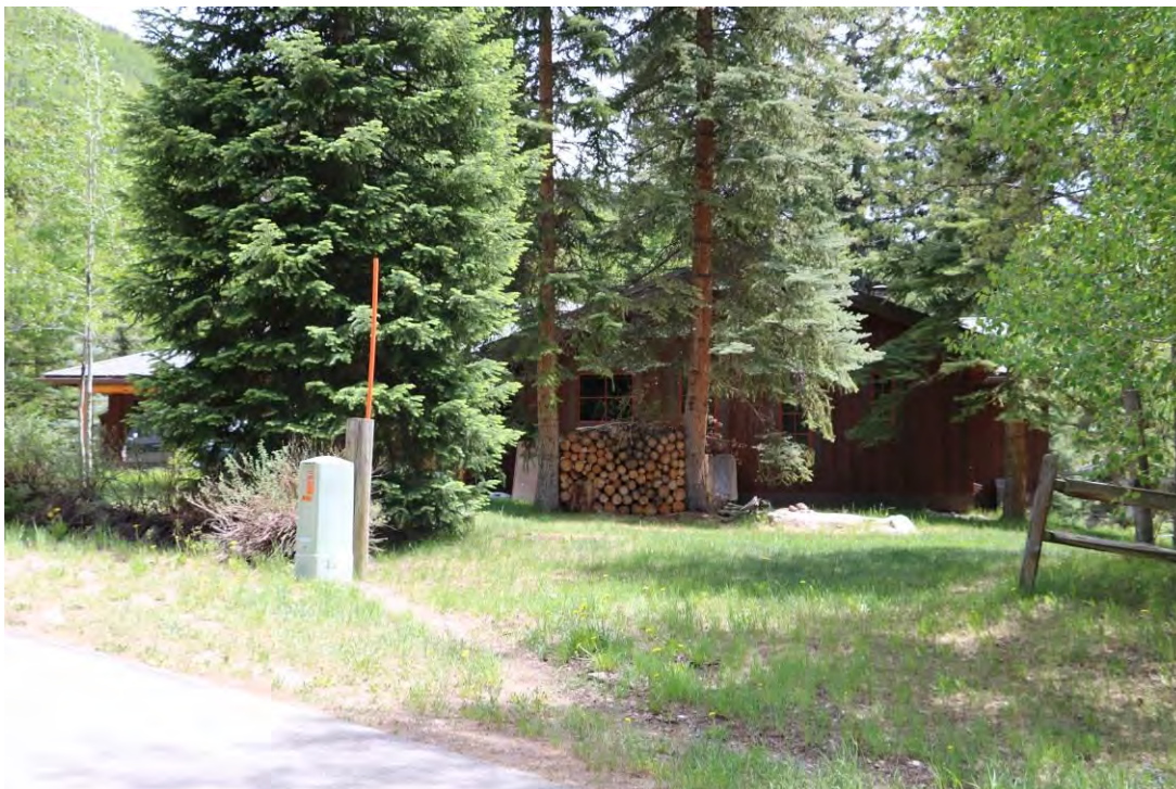
Front (northwest) elevation, view facing southeast.
