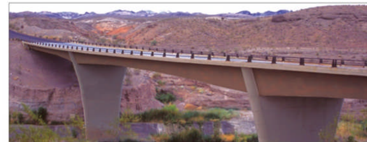
A | Bridges with simple forms, color, and shadow patterns exhibit an aesthetic contrast to the complexity of the natural landscape.
