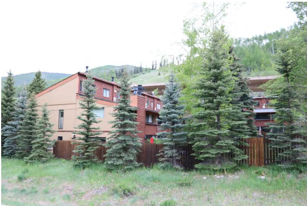
Overview of complex, view facing north.
