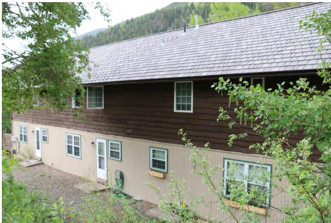
Rear (north) elevation showing the enclosed door for the third unit at right, view facing southeast.
