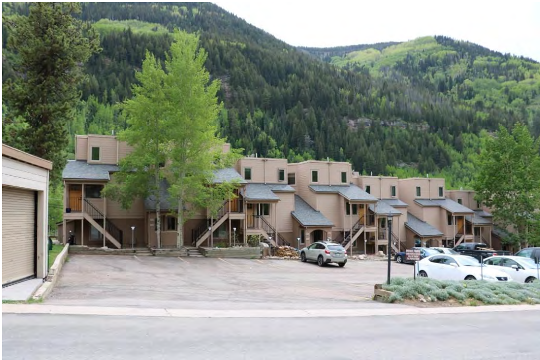
Northeast (rear) elevation and overview of setting, view facing southwest.
