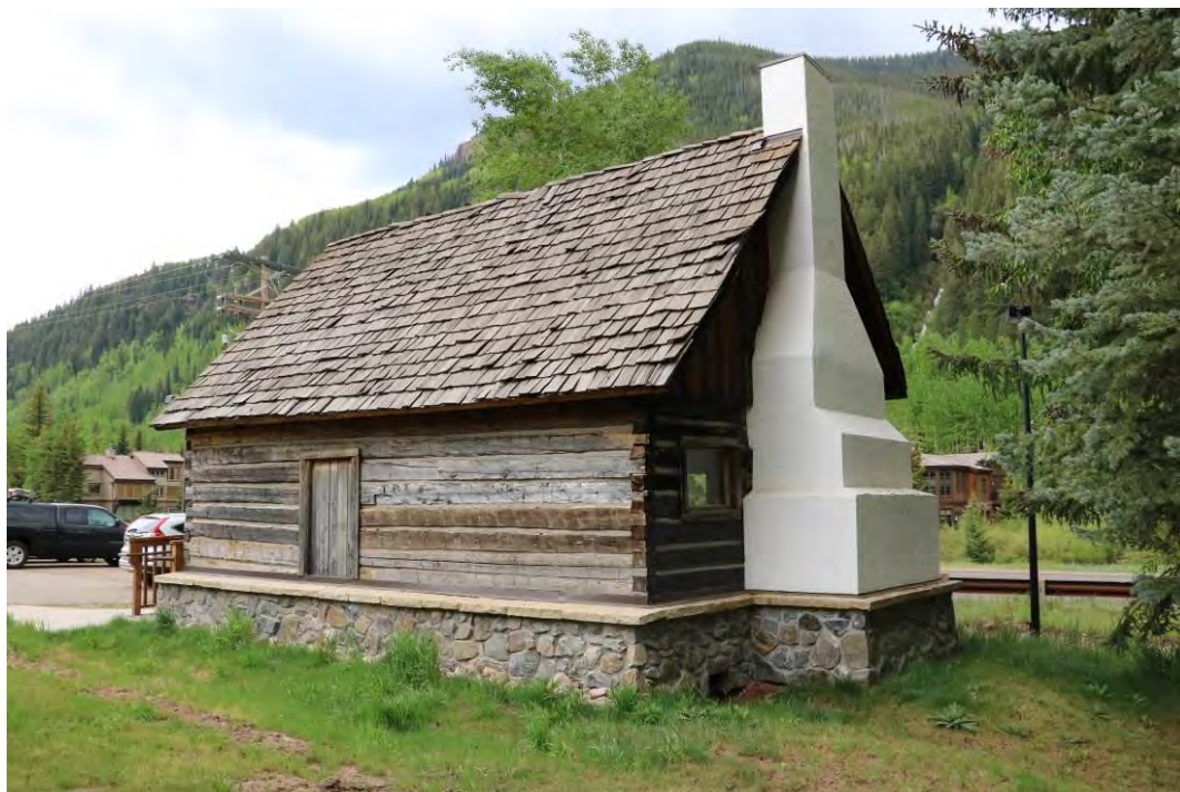
The rear (northeast) and side (northwest) elevations, view facing south.
