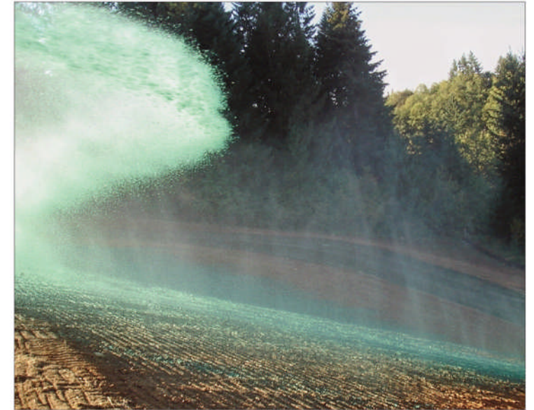
A | Mulching should be used to reduce dust and erosion impacts and promote successful revegetation.
