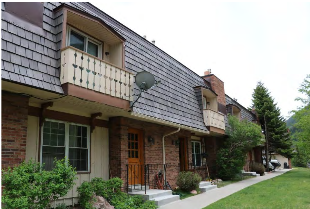
Detail of typical entryway, fenestration, and balconies on condominium units, view facing east.
