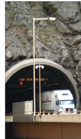
B | Light poles should be of an elegant and simple design with full-cutoff luminaire fixtures.
