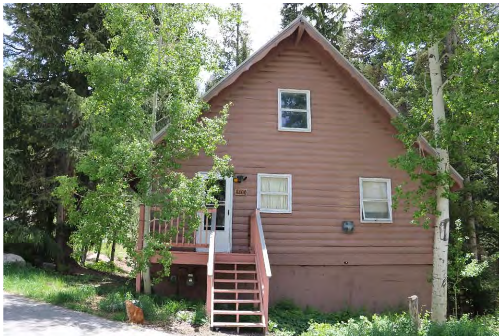
Overview of front (northwest) elevation and setting, view facing southeast.
