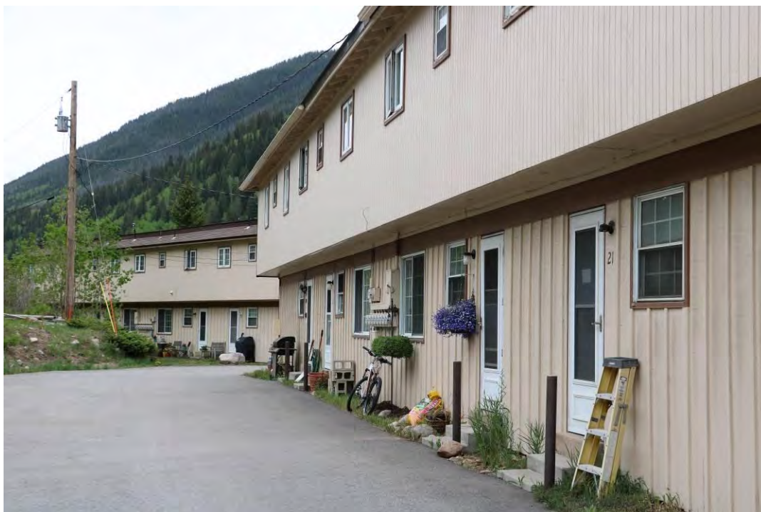
Rear elevations on typical buildings within the complex, view facing southeast.
