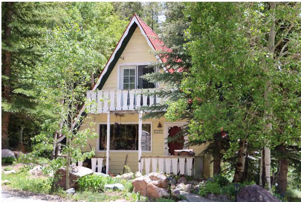
The front (northwest) elevation, view facing southeast.
