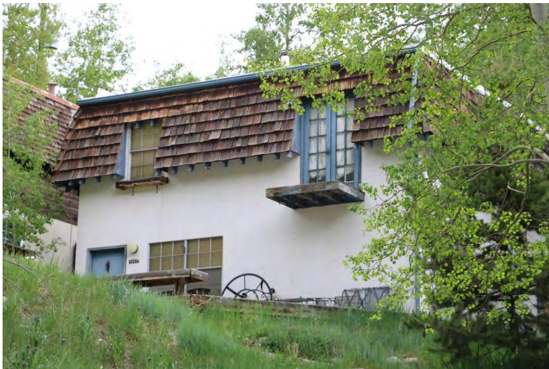
The front (southwest) elevation, view facing northwest.
