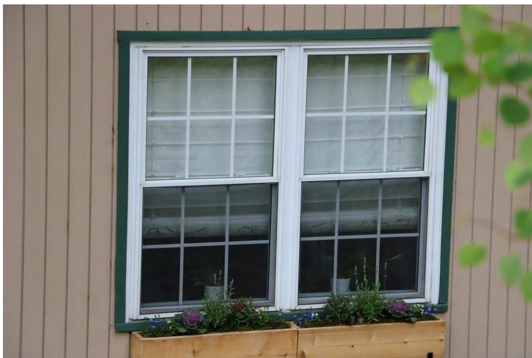
Detail of replacement, multi-light, vinyl windows, view facing south.
