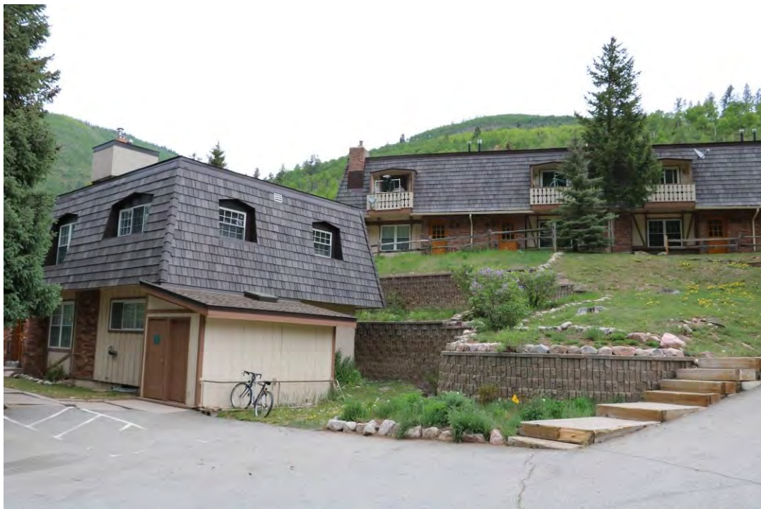
Overview of condominium complex, view facing northeast.
