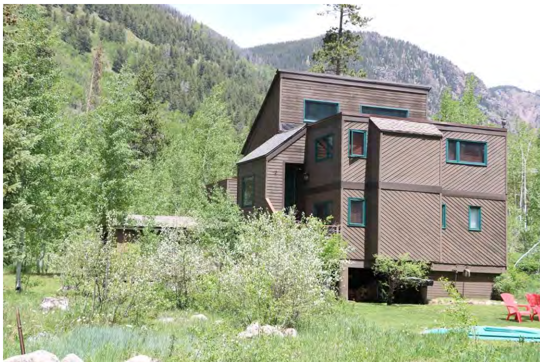
The front (northwest) and side (southwest) elevations, view facing northeast.
