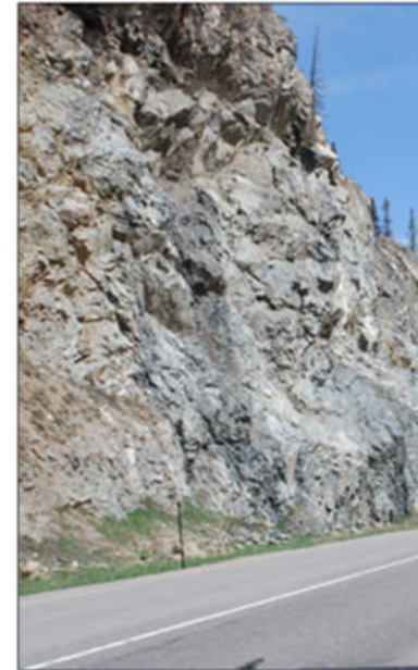
A | Color staining techniques may be used to blend new rock cuts with existing rock features.
