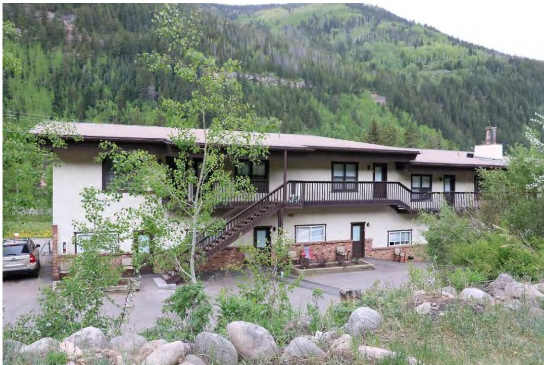
Rear (north) elevation, view facing south.
