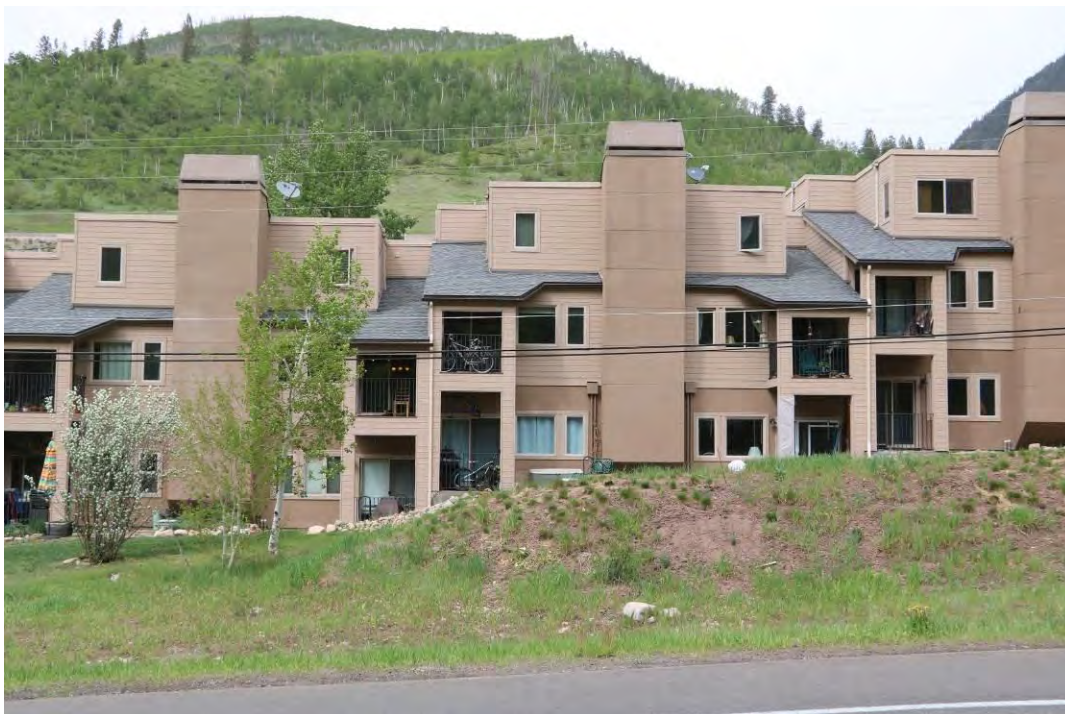
Detail of interconnected quadplex buildings, view facing northeast.
