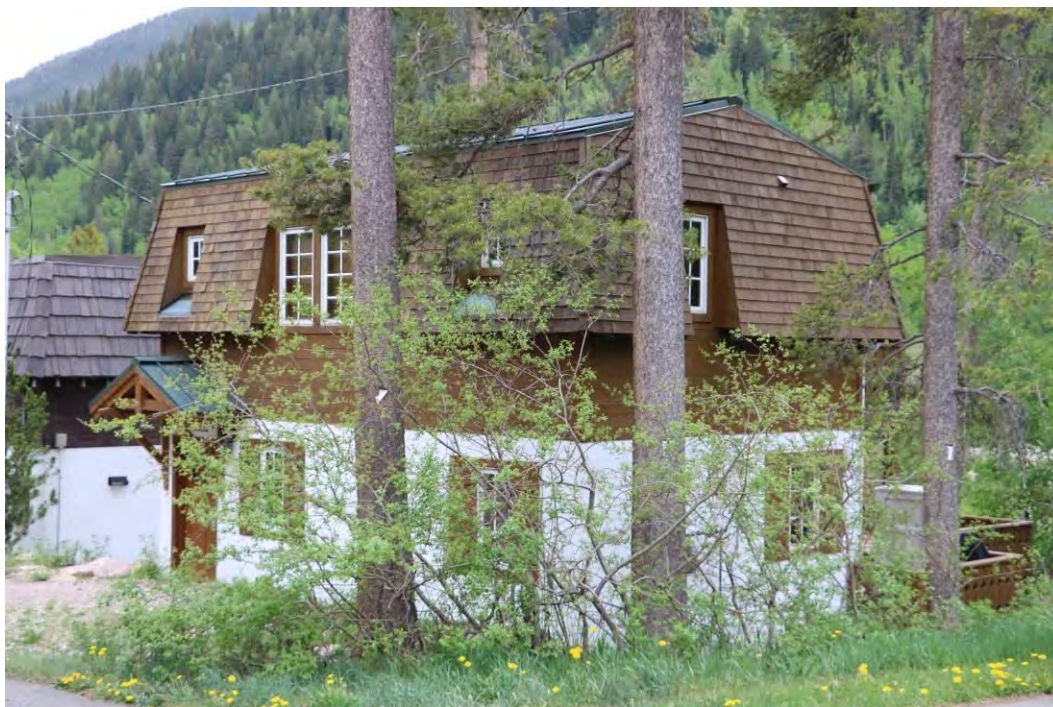
Front (northeast) and side (northwest) elevations, view facing south.
