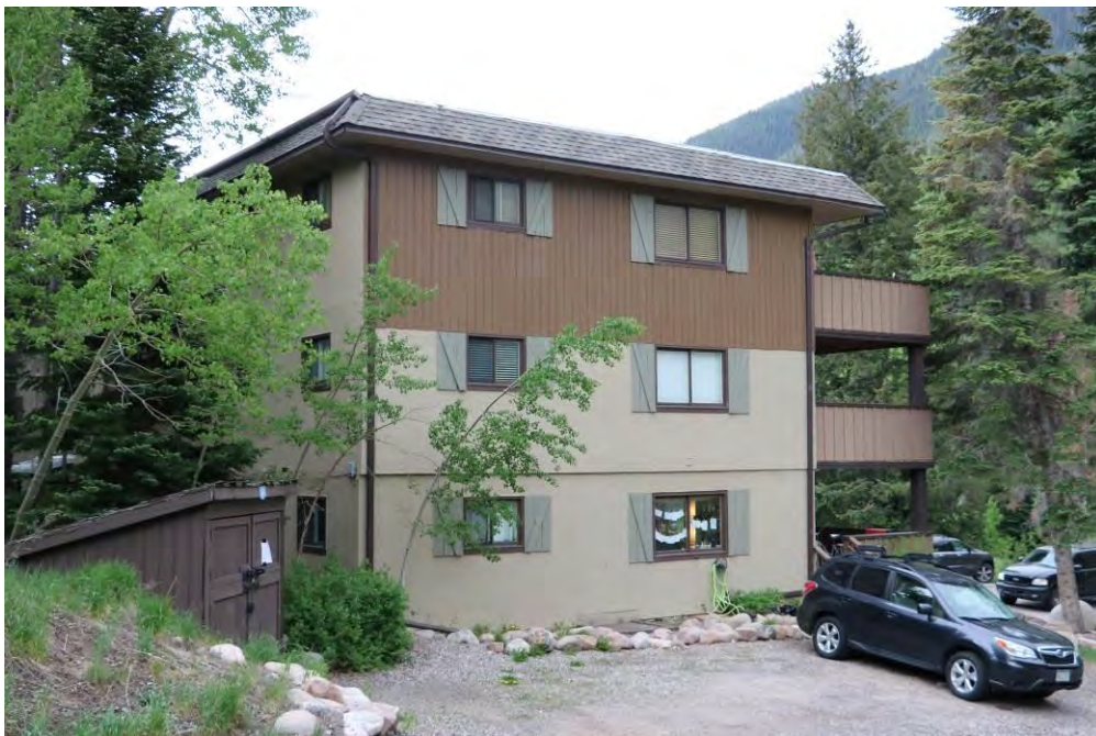
Northwest elevation, view facing southeast.
