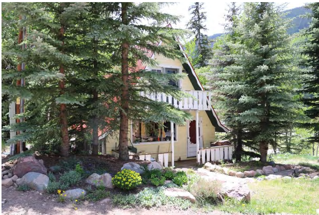
The front (northwest) elevation and setting, view facing south.
