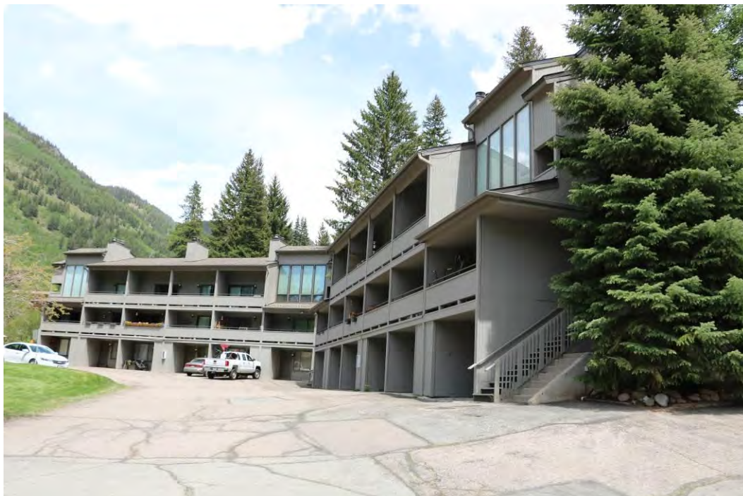
The front (northwest) elevations for both buildings, view facing east.
