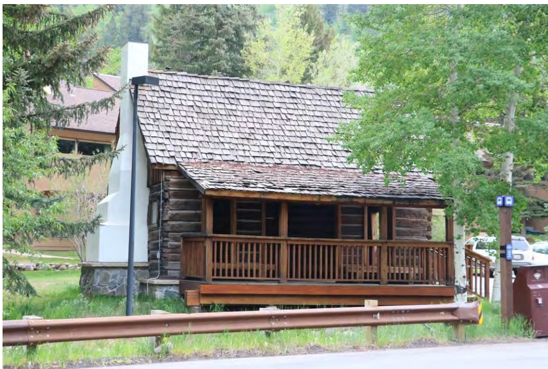
The front (southwest) and side (northwest) elevations, view facing northeast.
