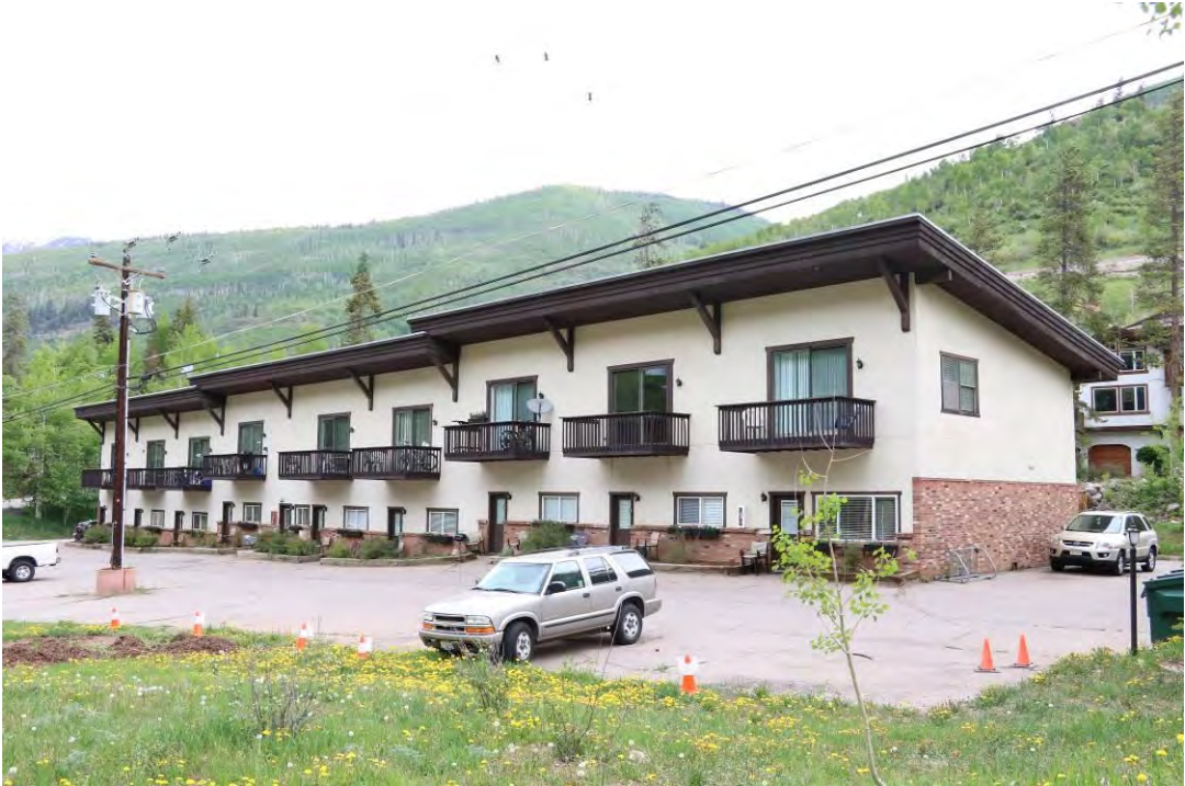
The front (south) and side (east) elevations, view facing northwest.
