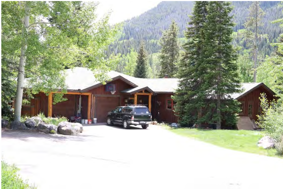
Front (northwest) and side (northeast) elevations with garage bays and main entrance, view facing south.
