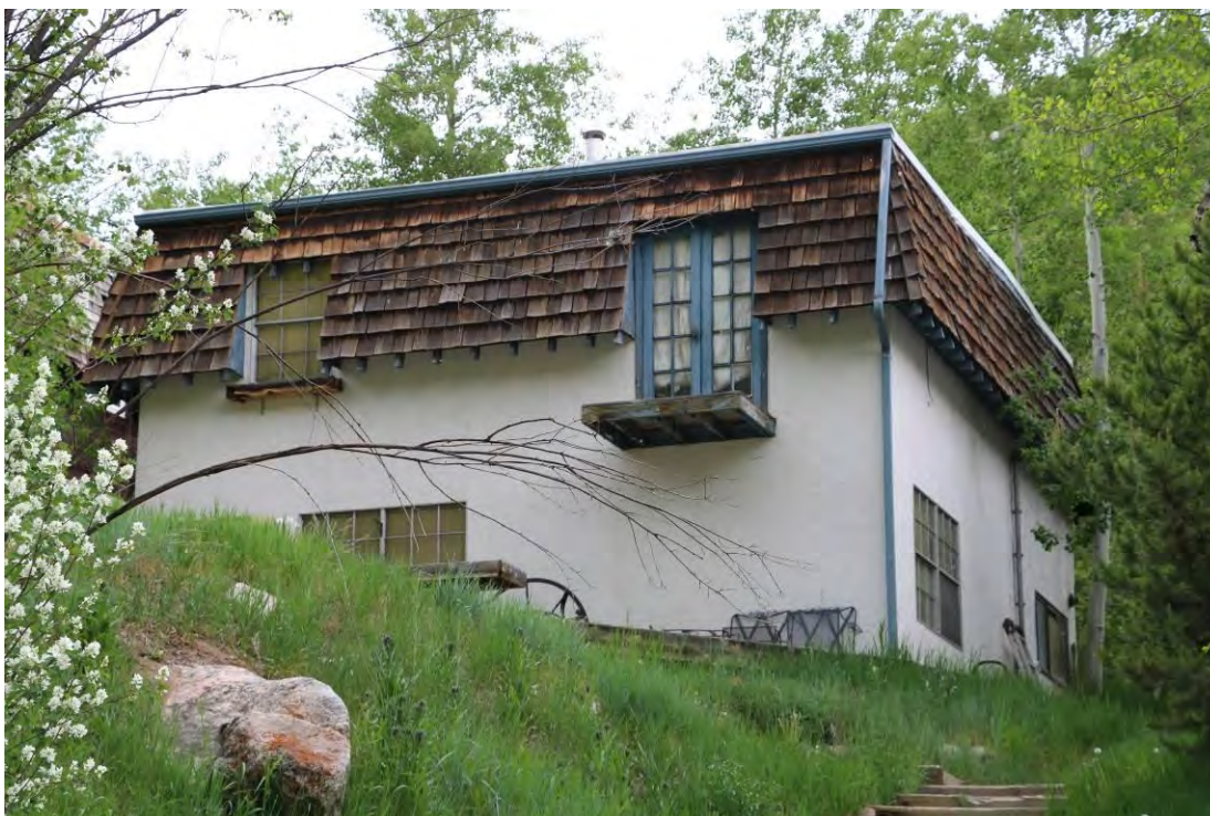
The front (southwest) and side (southeast) elevations, view facing north.
