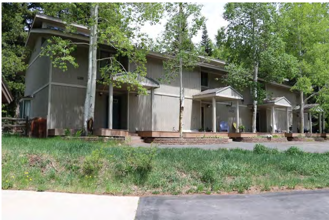
Front (southwest) and side (northeast) elevations, view facing east.
