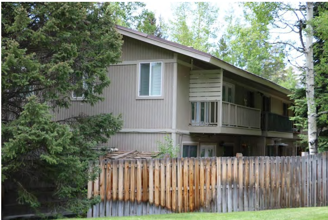
Side (southeast) and rear (northeast) elevations, view facing northwest.
