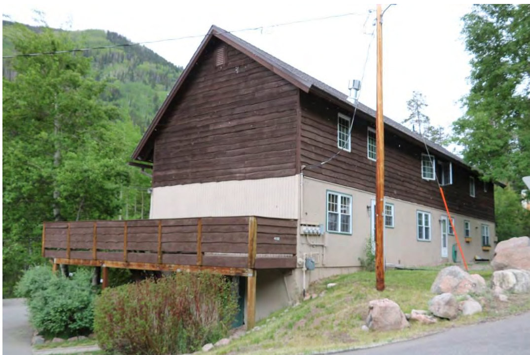
The rear (north) and side (east) elevations, view facing southwest.
