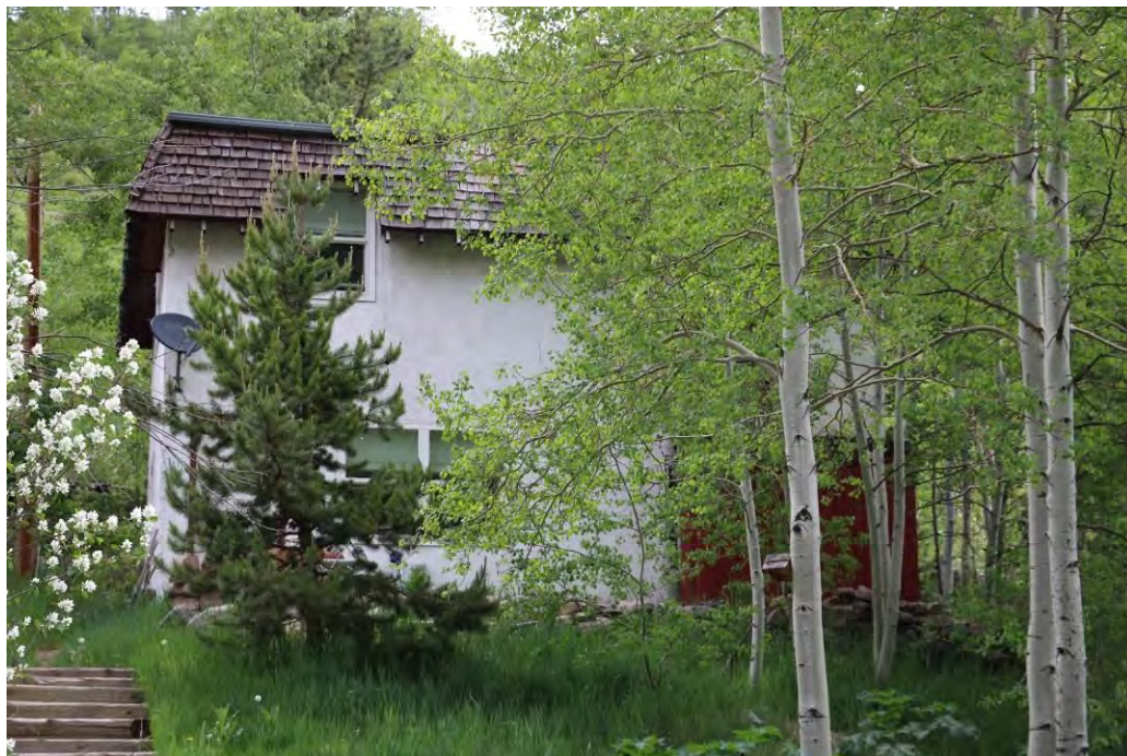
Overview of southwest (front) elevation and setting, view facing northeast. Small wood-frame shed is visible at far right, in front of the house.
