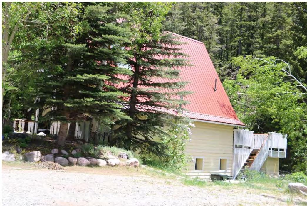
Southwest elevation and wood deck at rear, which extends around to southeast elevation, view facing east.
