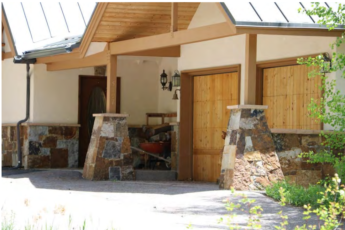
Detail of the front (north) elevation illustrating the range of replacement materials on the house, view facing southeast.
