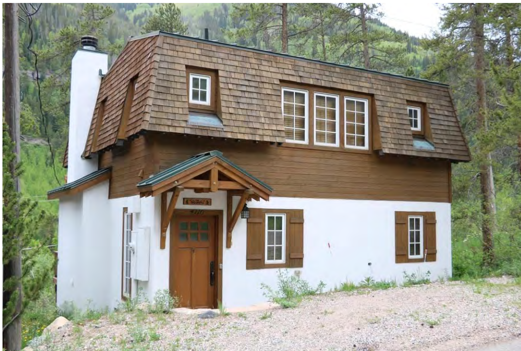
Overview of front (northeast) and side (southeast) elevations, view facing west.
