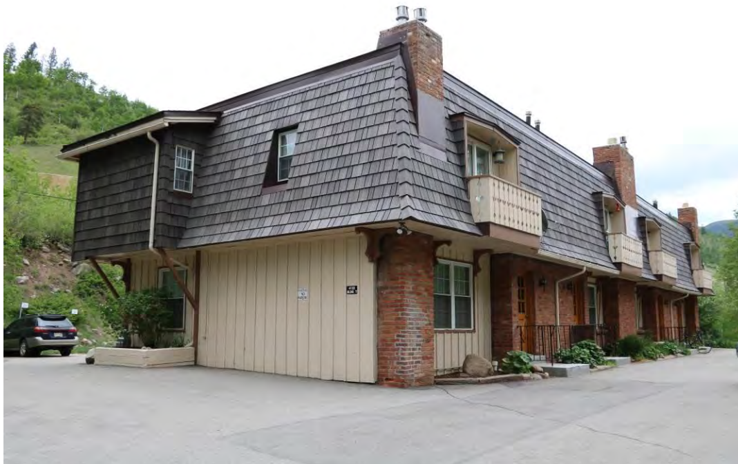
The front (southwest) and side (northwest) elevations of typical building within the complex, view facing east.
