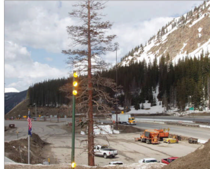
A | The approach to the Eisenhower Johnson Memorial Tunnel presents a cluttered and confusing mix of construction and maintenance uses to the
