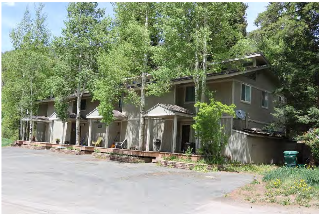
Front (southwest) and side (southeast) elevations, view facing northeast.
