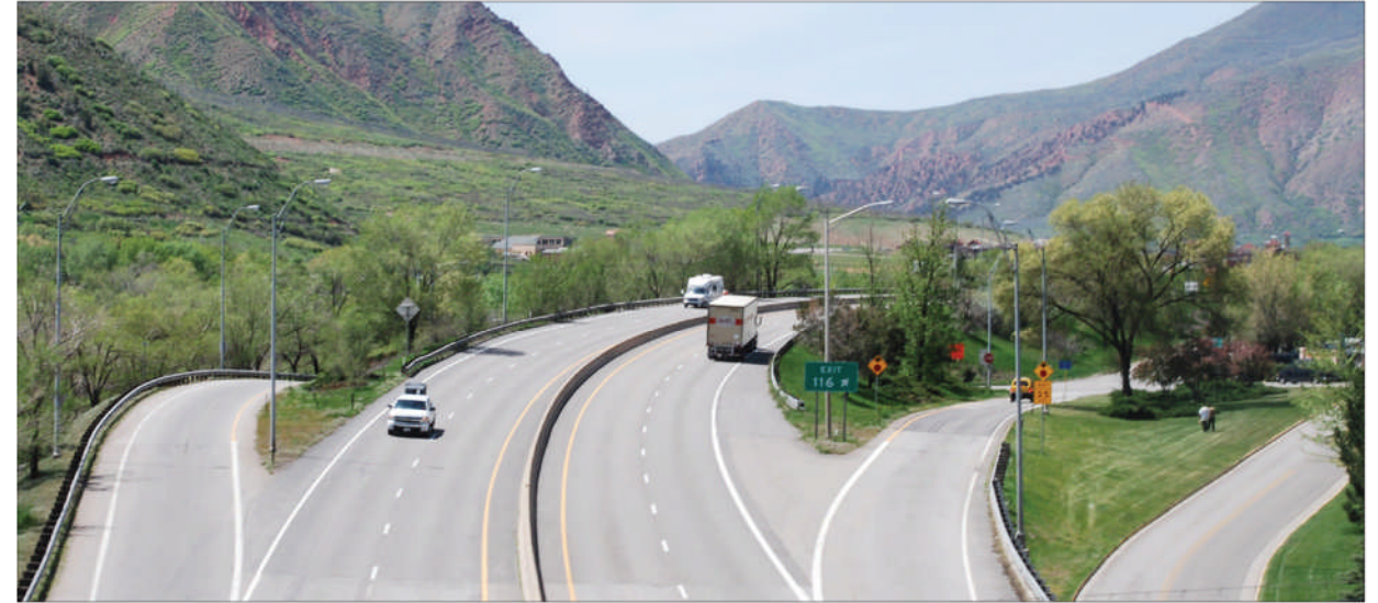
A | Interchanges should exhibit a compact design and include dense landscaping in open areas to create a transition from the transportation corridor to the community environment.
