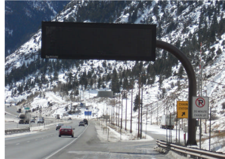
A | Single-arm monotube systems should be used.
