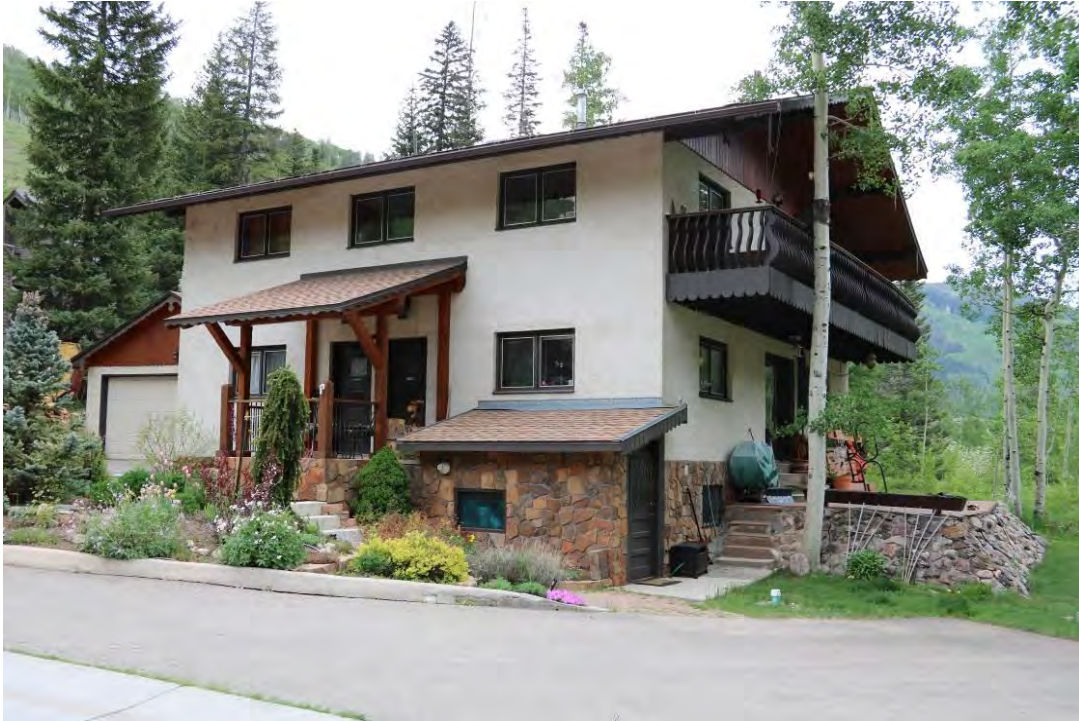
Front (northwest) and side (southwest) elevations, view facing east.
