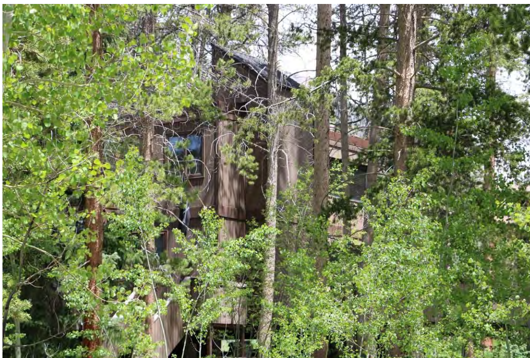
The front (west) and side (south) elevations, view facing northeast.
