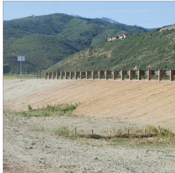
B | Utilize soil retention netting, mulches, and other revegetation techniques that improve the chances of successful re-establishment.
