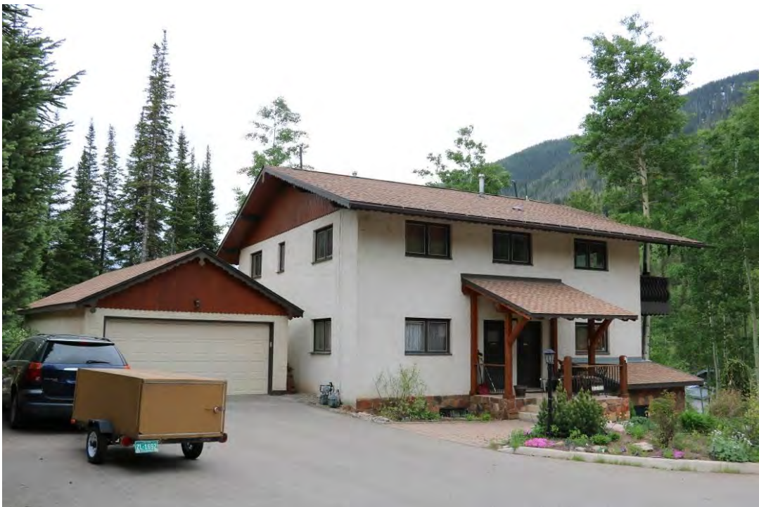
Front (northwest) and side (northeast) elevations and detached two-car garage, view facing southeast.
