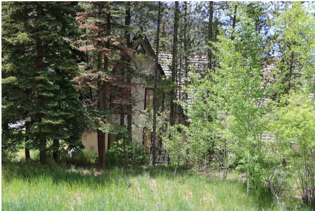
Side (east) elevation, view facing northwest.
