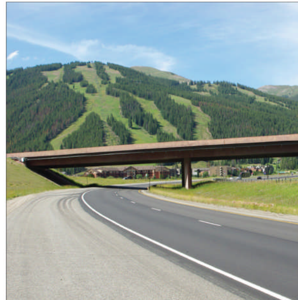
B | The bridge at Copper Mountain presents an aesthetic character with color, shadow, and box girder construction.
